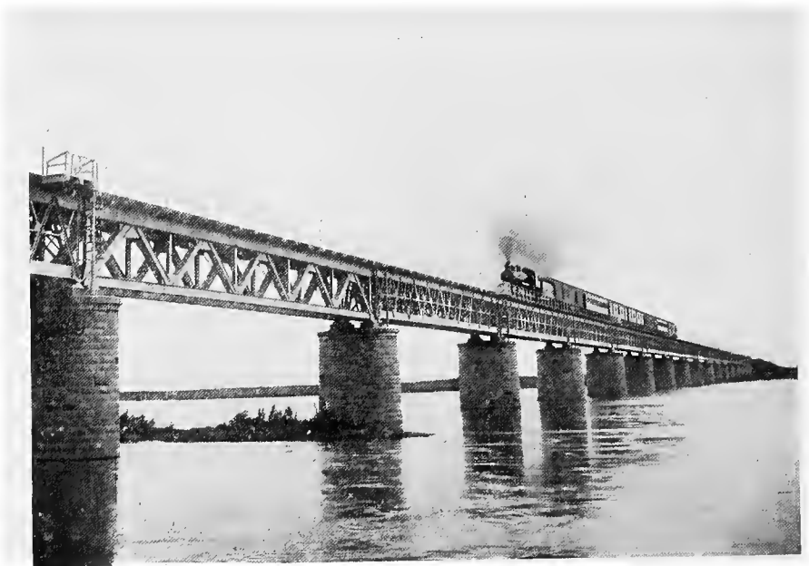
New South Manchuria Railway bridge built over the Hun River near Mukden
