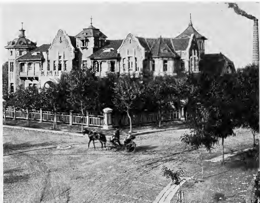
Fushun Club at the Fushun Colliery
