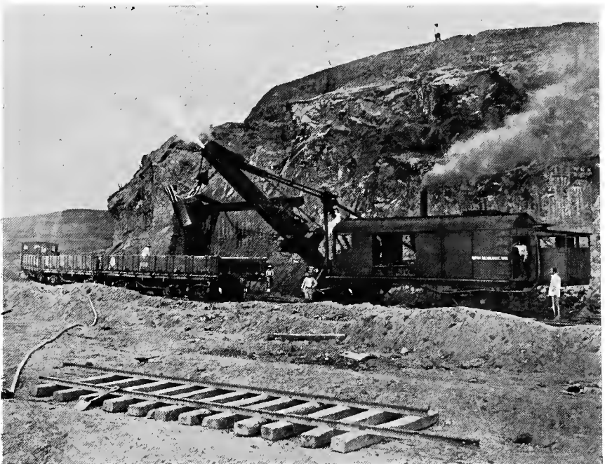
American steam shovel at work in the Fushun Colliery
