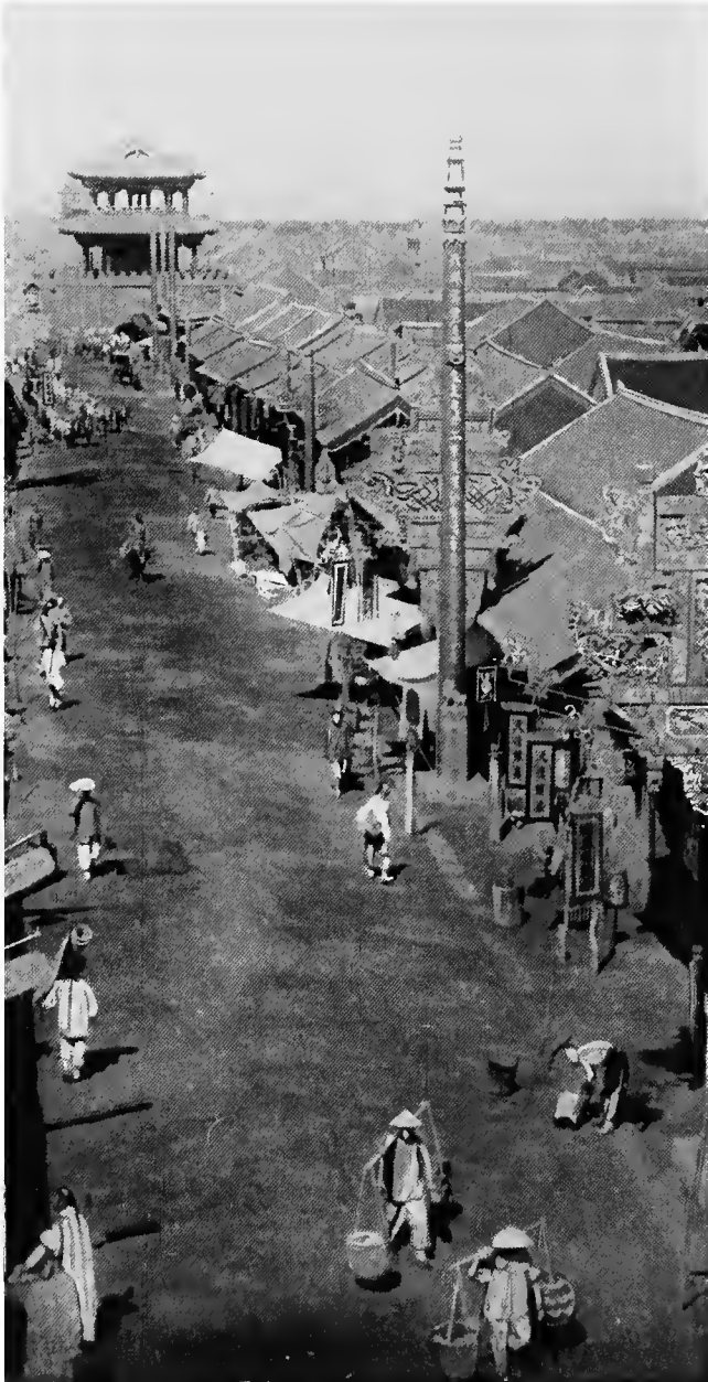
Looking down Ssu-Ping-Chieh toward the Bell Tower, Mukden
