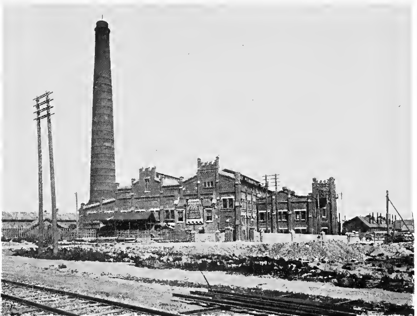
Electric light and power plant, Dairen
