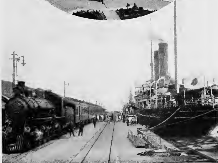
Facilities for quick travel connections are found at Dairen
