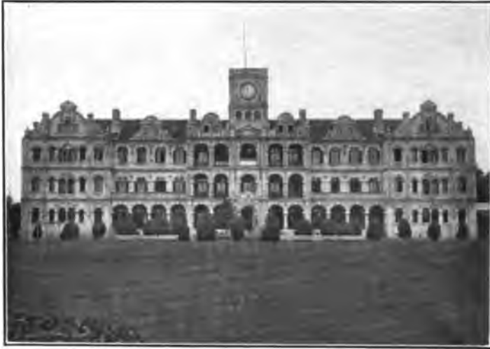
TECHNICAL DEPARTMENT BUILDING—SHANGHAI Showing the Progress of Education in the Celestial Empire
