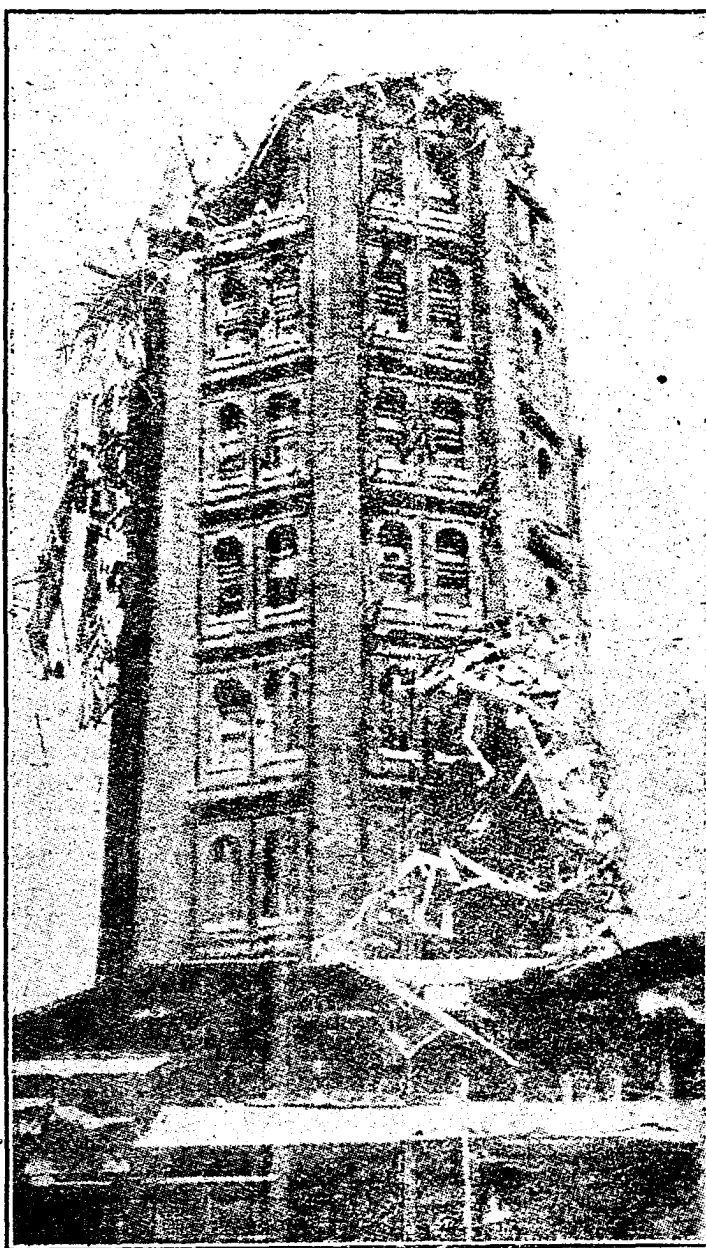
REMAINS OF THE 12-STOREY PAGODA AT AKASUKA PARK, TOKIO.
